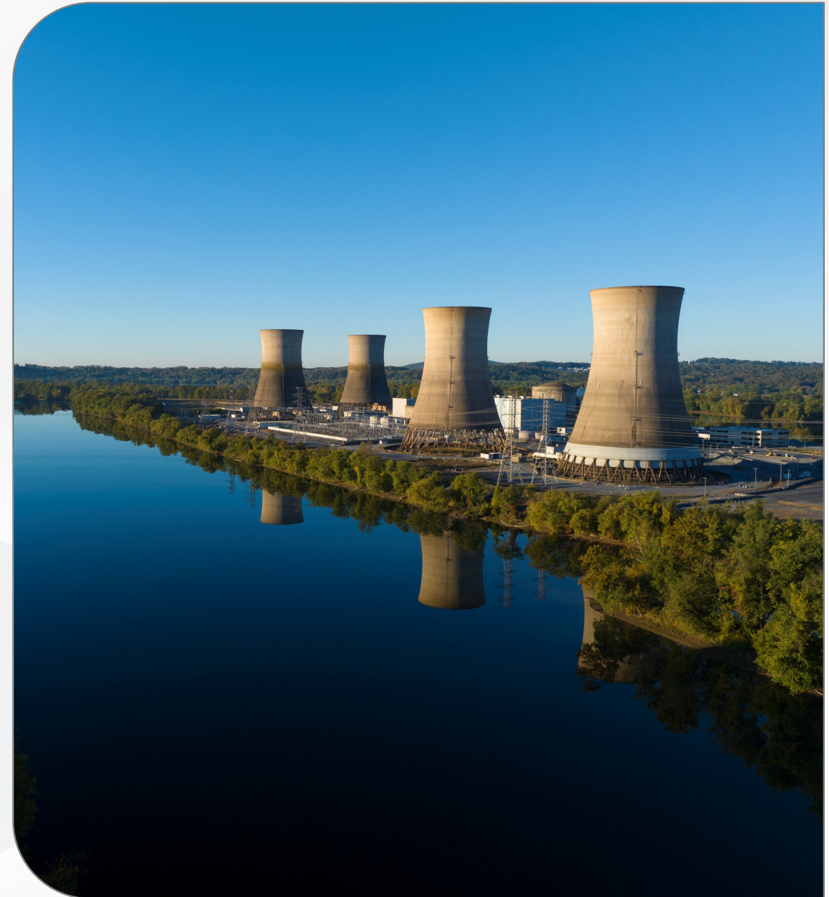
Crane Clean Energy Center
