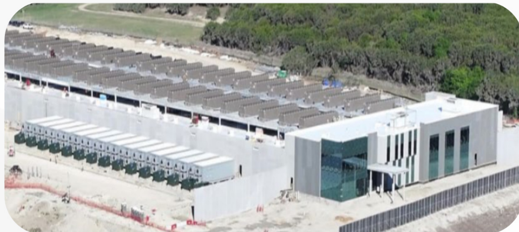
Data Center at Thad Hill Energy Center
