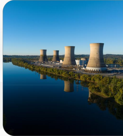
Crane Clean Energy Center
