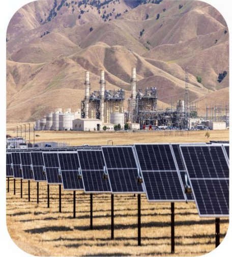
Pastoria Solar Project, CCGT, and battery storage colocation
