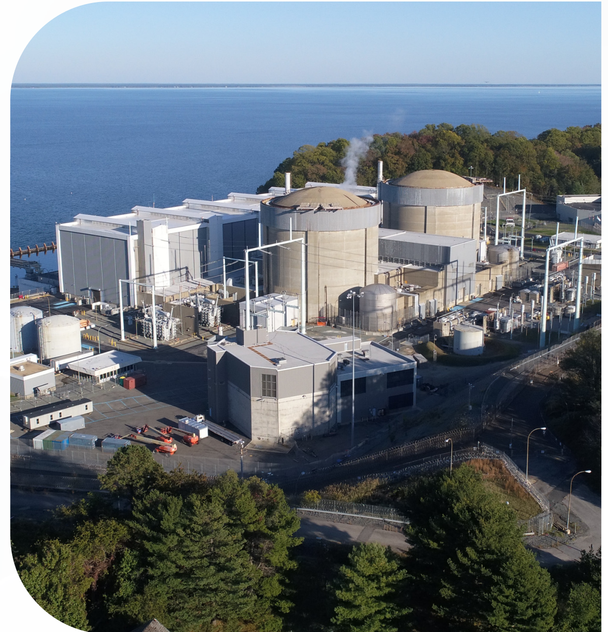
Calvert Cliffs Clean Energy Center
