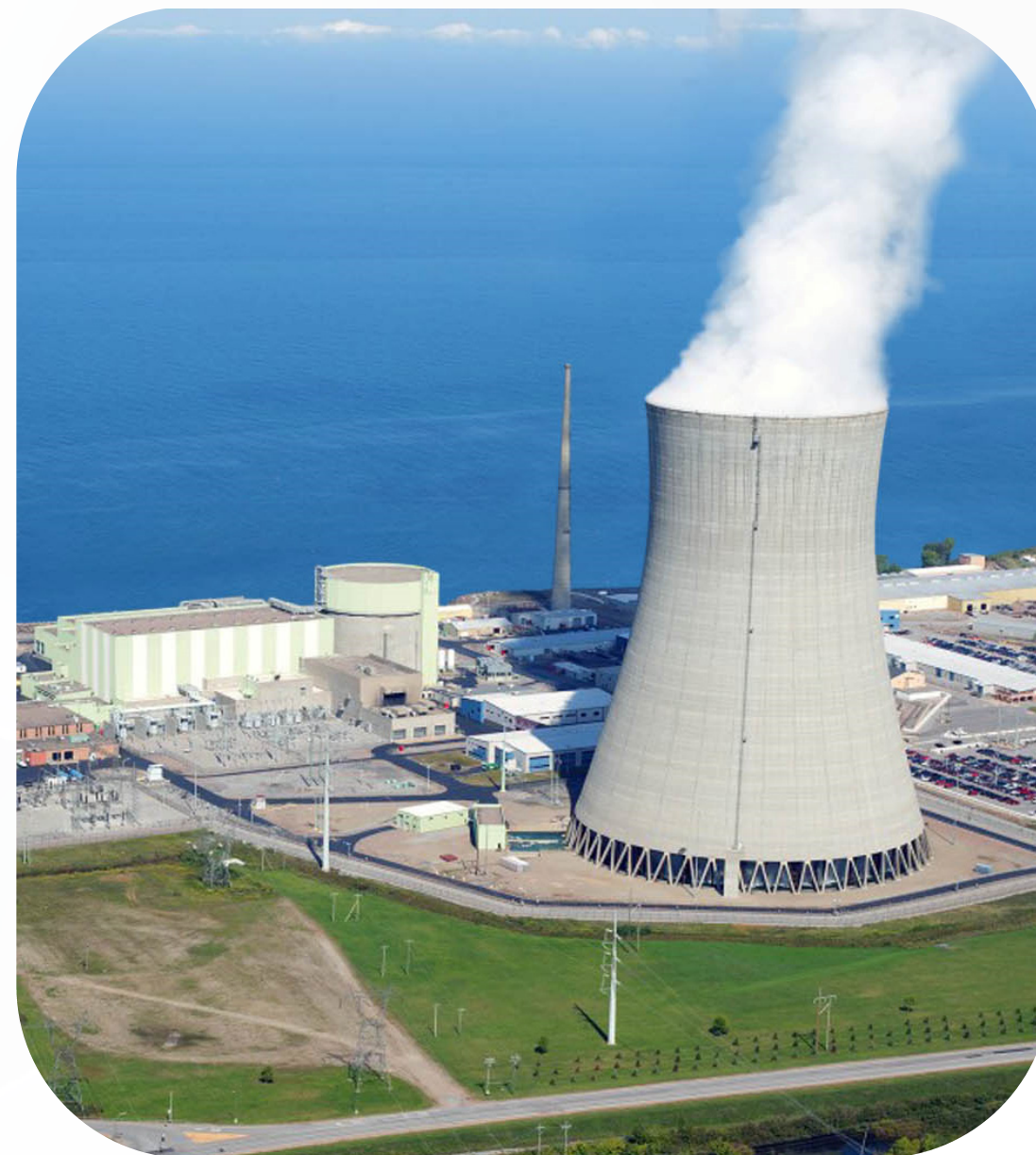
Nine Mile Point Clean Energy Center
