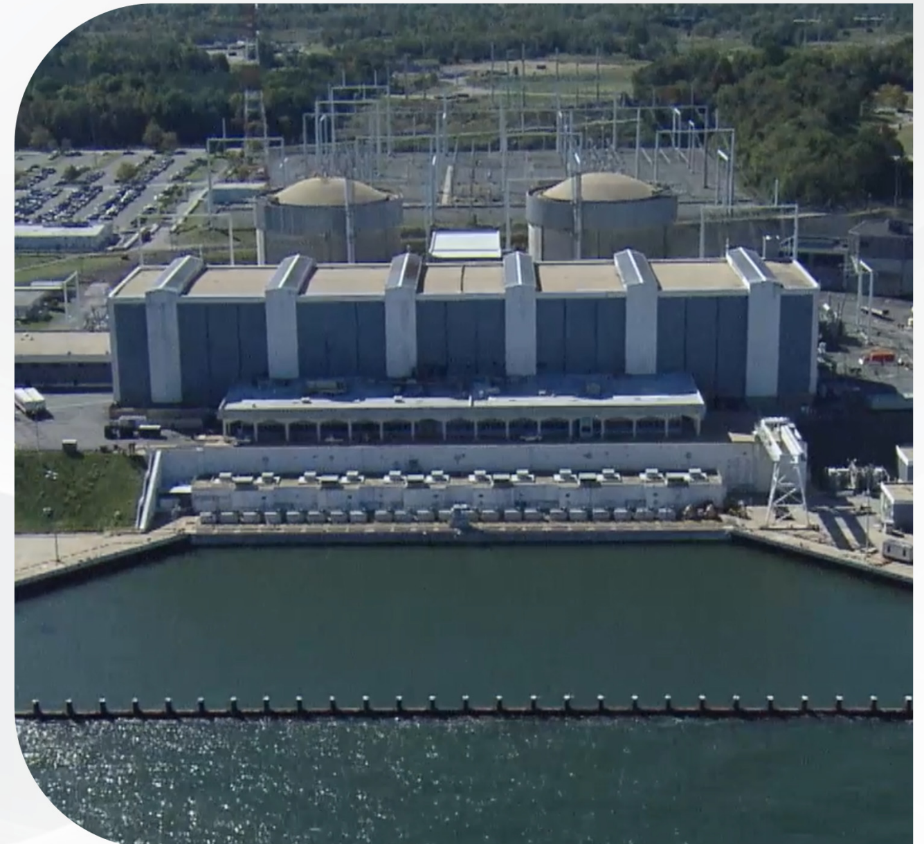
Calvert Cliffs Clean Energy Center
